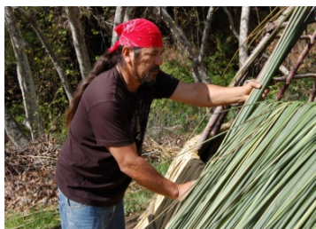
Mati Waiya applies newly harvested tule reed bundles to the willow frame of an 'ap - traditional Chumash house
